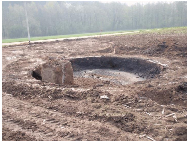
Fig. 32: Uncovered shaft head of HAM II on 14.04.2016
